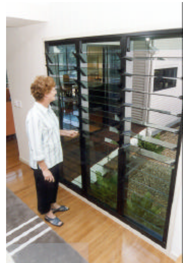
Louvres provide cross-ventilation to overcome the summer heat.
