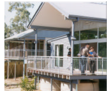
Rainwater tanks were installed to achieve greater water efficiency.
